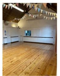
restored, sanded and sealed. Removal of the furniture in the hall and sink unit in the toilets revealed areas of rotten floor planks which have also been replaced. The new sink unit is in situ and further work to 'make good' in the toilets will happen over the next few weeks. Our new chairs are also imminent, so our April Pop-Up Café will be a great opportunity to sit more comfortably and see the transformation.
